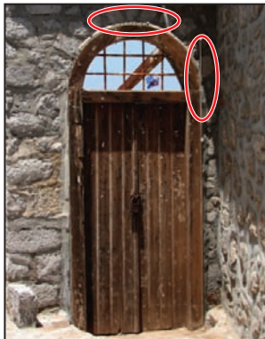
The completed curve.
